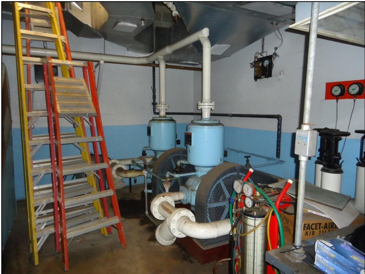
Figure 11. Room 171, Vacuum Pumps
